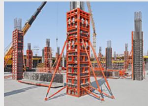
Column Formwork
