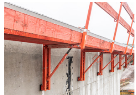
VGK Flex is designed for forward and backward sloping walls.
