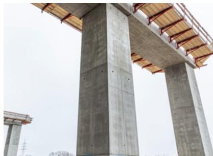
As working platforms, VGK Console Brackets provide safe and convenient working conditions.
