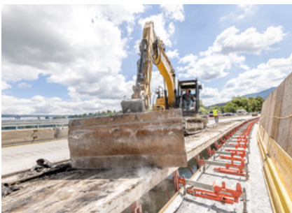
VGK Console Brackets ensure safety underneath the bridge and during work operations on the bridge.
