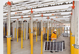
Slab Formwork
