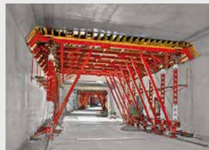
Tunnel Formwork
