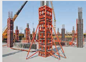
Column Formwork
