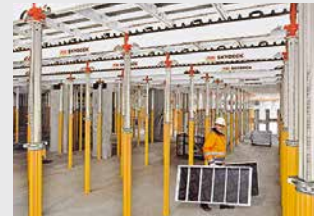
Slab Formwork
