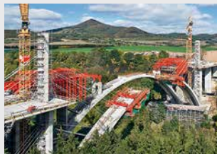
Bridge Formwork
