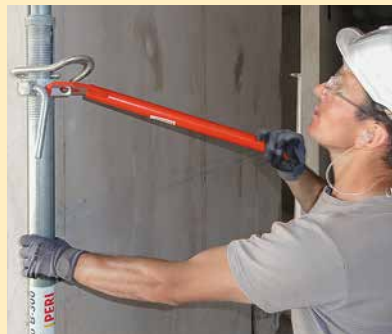
Ergonomic operations through offset wingnut spanner.
