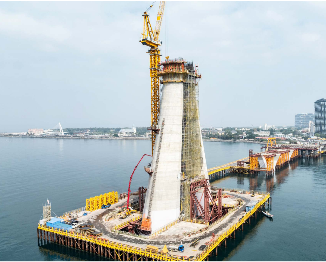
Danjiang Bridge, New Taipei, Taiwan
