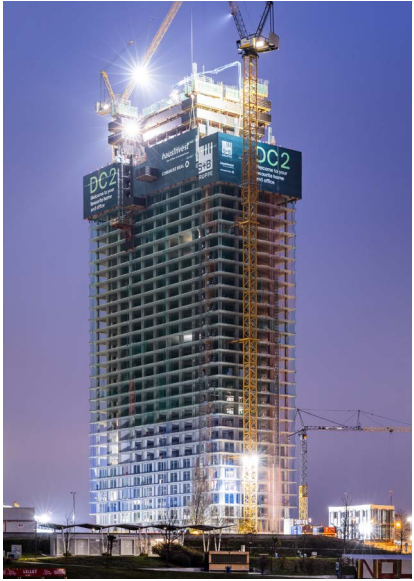
By using the new RCS MAX Mobile Hydraulic System, it was possible to climb two climbing platforms into the next section using rail guidance.
