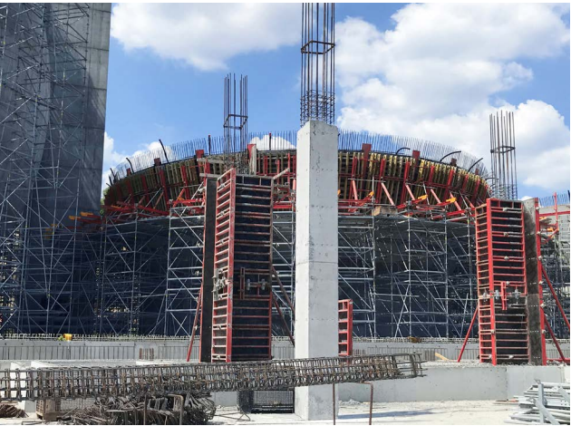
With PERI Formwork and Scaffolding Systems from a single source, it was possible to construct the complex clarification plant in an efficient manner.
