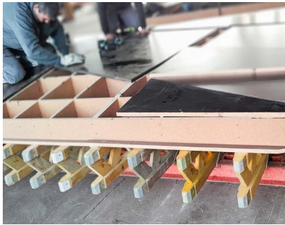
A variety of panel types were used for the special-purpose formwork in order to meet the architectural requirements in the best possible way.
