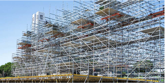
The PERI UP Scaffolding Kit was used to create multiple access points to support the safe execution of the choreography planned for the event.
