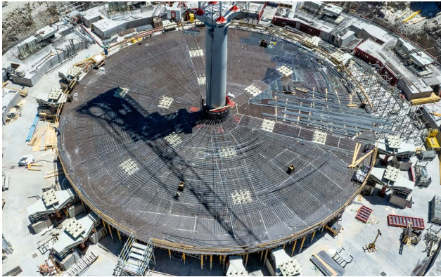
The base in the centre of the ELT was built quickly and flexibly with the aid of MULTIFLEX Girder Slab Formwork.
