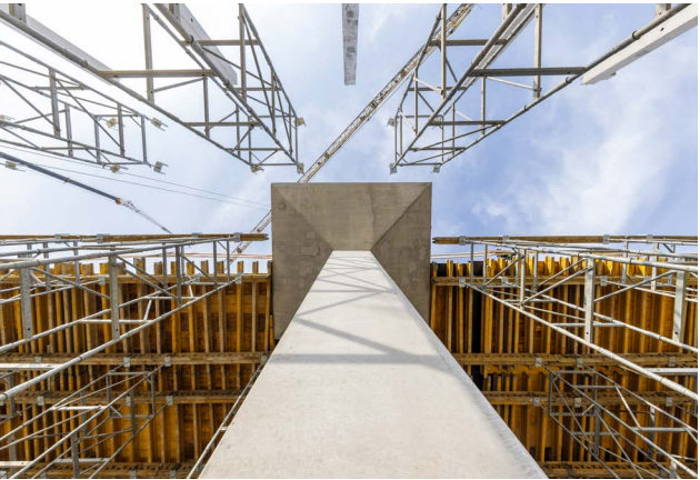
A combination of several formwork systems provided the central building block for the prefabricated columns with bases in the second and third sections of the hall.
