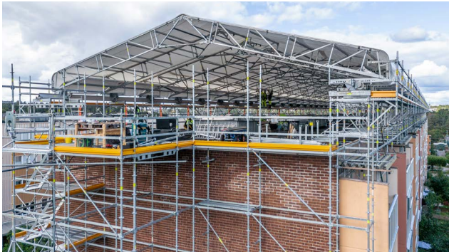
The PERI UP LGS 75 is a slender weather protection roof that was able to bridge the span width of 13 m with ease.
