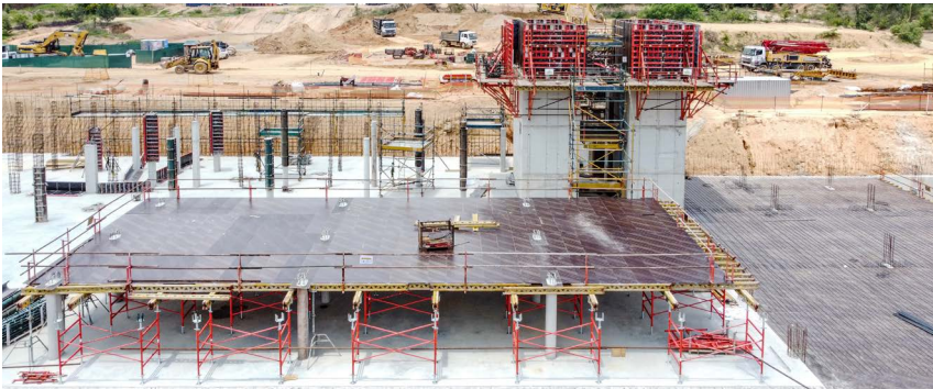
Pre-assembled slab tables were used to ensure efficient production of the slabs, thus increasing productivity on the construction site.
