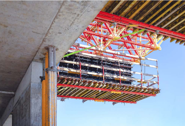
The VARIODECK Steel Waler Slab Tables were very well suited to the project, as these large slab tables facilitated a short concreting cycle.
