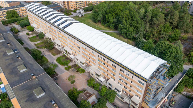
The logistics of transporting the work materials upwards was solved by using a working platform made of system components and a material lift.
